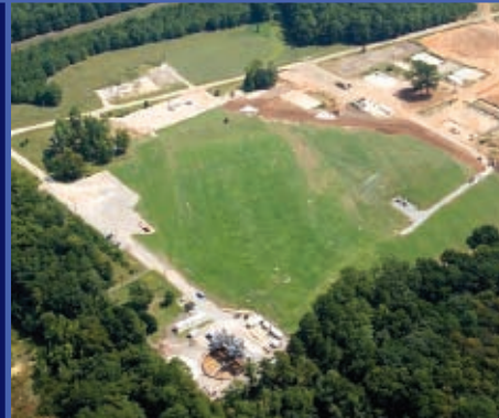
T Area After Demolition
