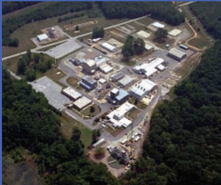
T Area Before Demolition
