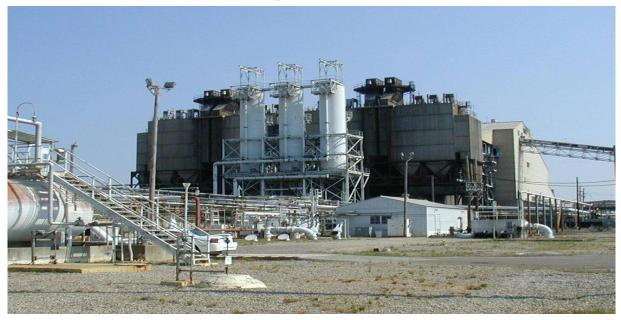
The existing D-Area Powerhouse was built in 1953 and provides steam to nuclear and industrial activities in F-, H-, and S-Areas. It is a co-generation facility and provides approximately one half (20 MW) of the Site's electrical demand.
