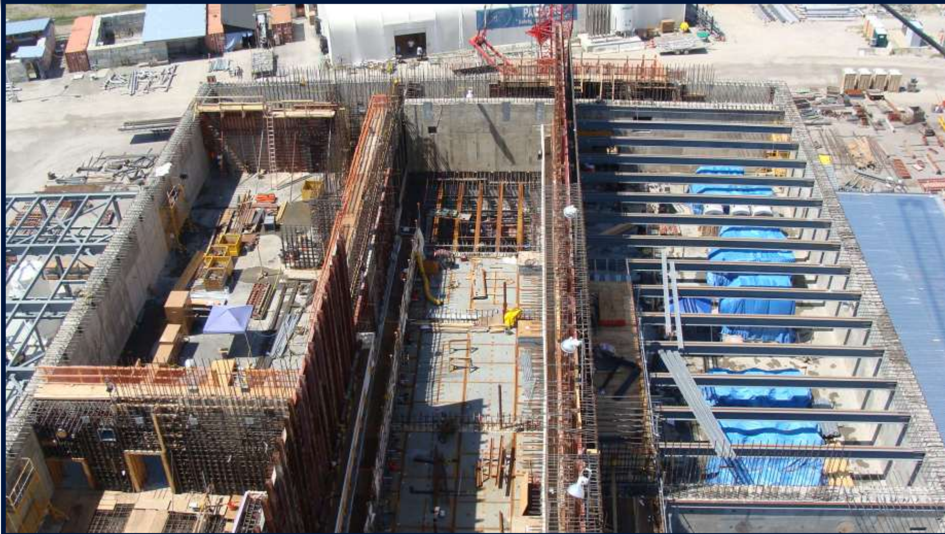
Operating Deck Over ASTA, Facing West
